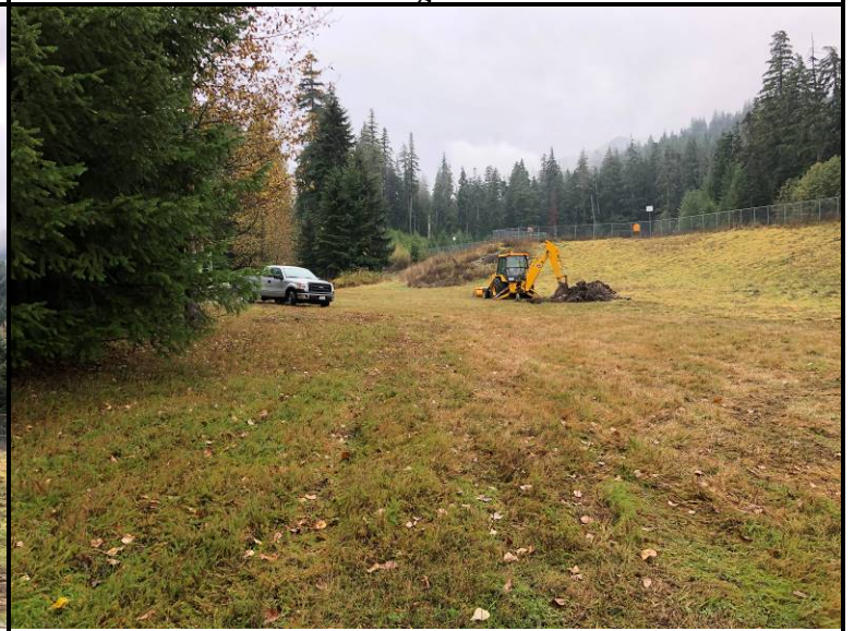
View of conditions looking south
