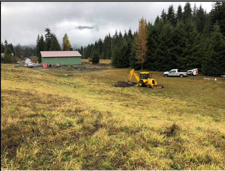
View of site conditions looking north
