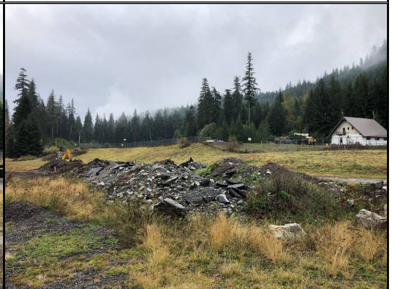
Stockpiles of fill soils and construction debris in northern portion of the proposed improvements area
